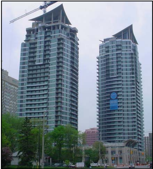
Two new apartment towers in the City Centre Planning District.
