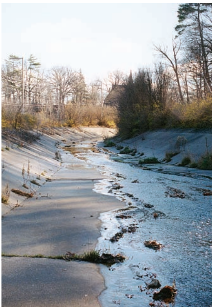
Old design, concrete-lined banks for stabilization along Sawmill Creek
