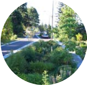
Stormwater swale, Portland OR
