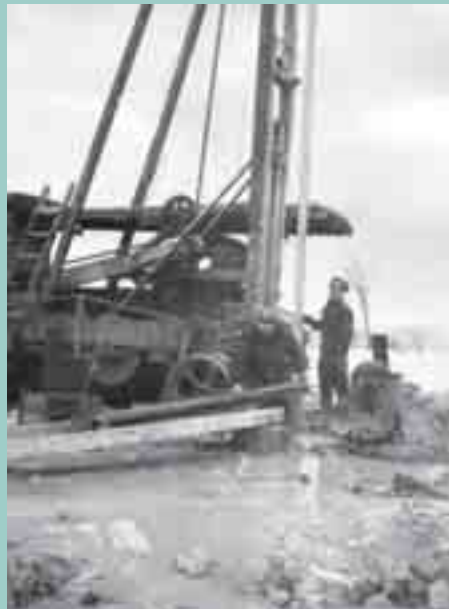
◀ Well testing for capacity - 1948 (Rogers Communications Inc.)
