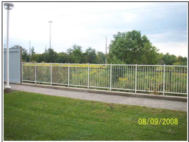
Photo 6: Acorn Place Apartment Building – View 2 South
