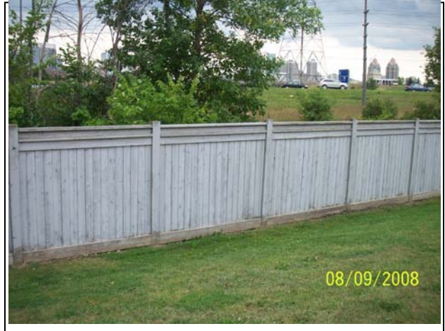
Photo 4: Acorn Place Townhouses – View 2 South
