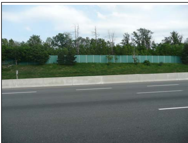
Photo 17: Earthen Berm + Noise Wall (south of Highway 403 between Winston Churchill Boulevard & Glen Erin)
