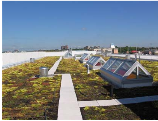
Figure C6.5 Green Roof
