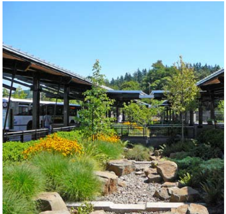
Rain gardens and bio-swales are examples of ways to treat surface storm water within a development area.
